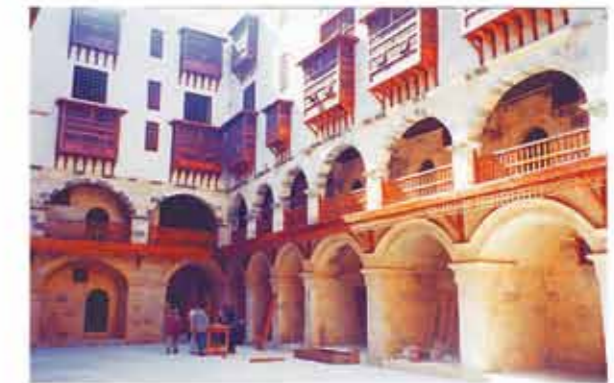
Wekalet Bazaraa following restoration
