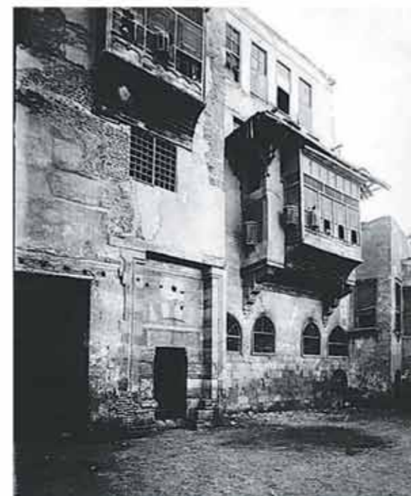
Beit El-Razaz before restoration
